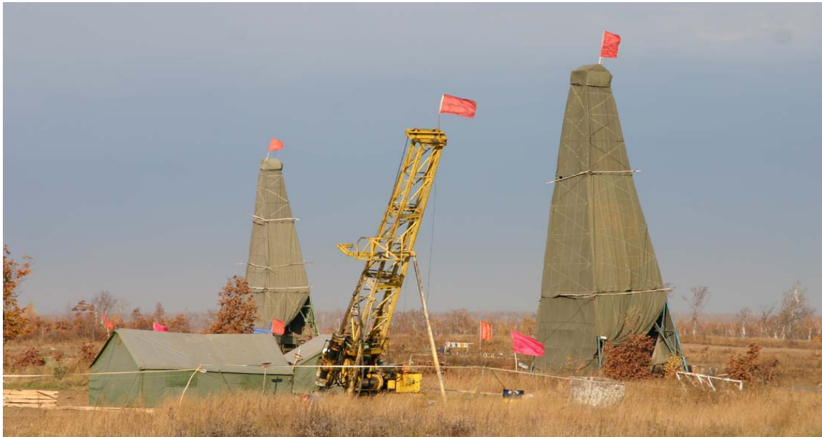
Figure 1 – Sinorex rig (yellow) with HLJBGMR rigs in the background
